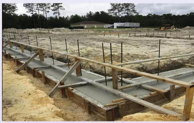
**STEP 2:** When the completed building materials and components arrive on site from the factory, they will be parked over the footings, while the foundation is being created. Then after, precisely maneuvered into place against the retaining wall by the setup crew using a Translift.
