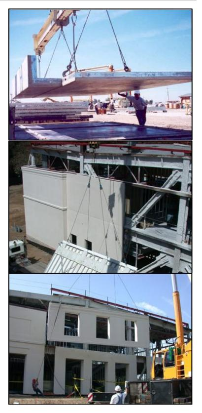
Lifting the Panels out of the Beds to be stacked on the trucks for transportation.
