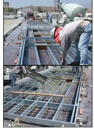
Metal stud framing, welded wire fabric and shear connectors laid out on casting beds.
