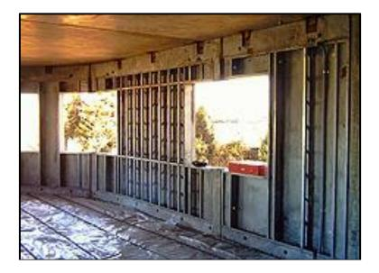
An example of interior view after erection, prior to rough-in and insulation.
